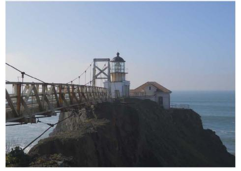
of the bridge. Both the western bridge tower and anchor block are founded in the diabase. Based upon visual observations at the surface and examination of rock core from the exploratory boring. The diabase is weathered, hard, and moderately fractured. These features are creating wedge failures resulting in oversteepened slopes and potentially unstable conditions of the bridge.
